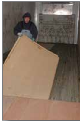
Plywood floor covering
